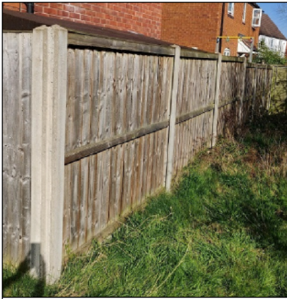
1.8m high concrete post and timber fence
